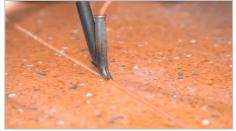
1.1.2 Welded seams must cool to room temperature before trimming in two steps, rough and fine trimming.
